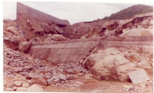
Chute Spillway of Bhagalati Irrigation Project
