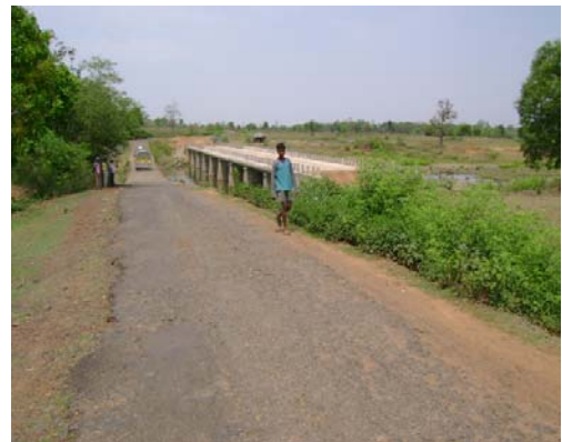
Bridge over river Bankal at 1 st km on Banki-Badamitalia road completed without construction of approach road
